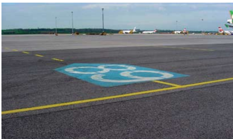
Above, new “alternative aircraft stand” taxi lane markings. Below, old “stand direction” marking.
