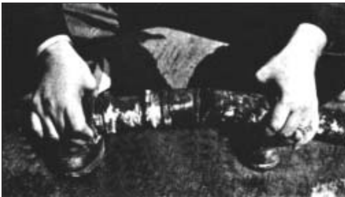
Figure 2. Where fuel hose burst. Note short section of rigid iron pipe which placed strain on hose when reeled.
