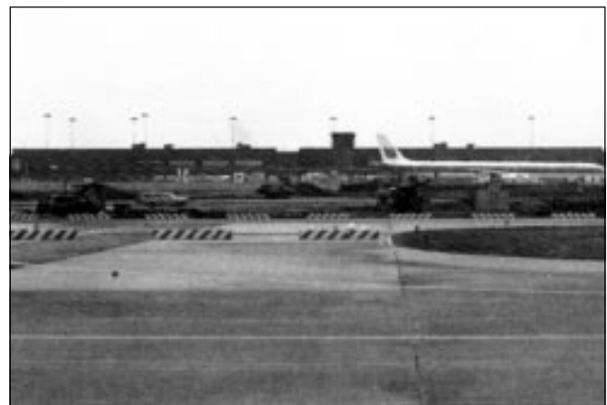
Weighted, low-profile vehicle barriers (cross-hatched) are less apt to damage passing aircraft or to be blown over by jet blast than barrel-shaped highway barriers.
