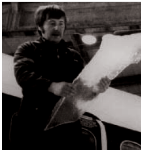
A mechanic holds a sheet of ice taken from the wing of the Finnair DC-9 that aborted a takeoff at Helsinki-Vantaa Airport in 1985 after flexing wings on the uneven runway broke the ice free, and it was ingested into the engines.
