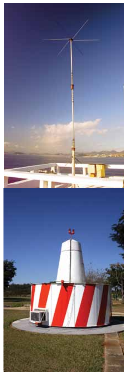
Photos: © Brazil Air Traffic Control
