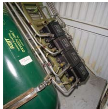
The FAA technical center is evaluating wireless smoke detectors (top) and flow-through air analyzers (bottom) in the cargo compartments of a Boeing 727 freighter.
