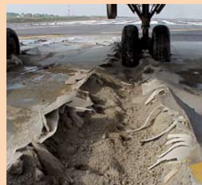
Port Authority of New York and New Jersey
